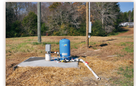
▲ This well has a concrete pad to help minimize the risk of contamination.
